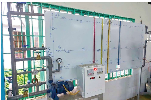
Figure10: The equipment system after installation
