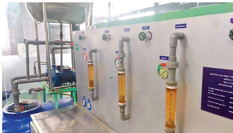
Figure 5. Pump-connection experimental equipment of IUH [1]
